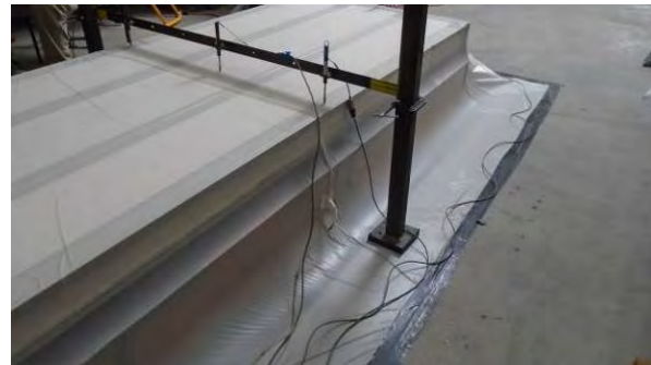
Photo 4: Transverse Load Set Up
