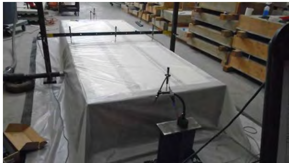
Photo 3: Transverse Load Set Up
